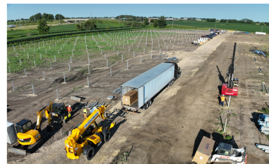
Post Pounding and Racking Preparation
